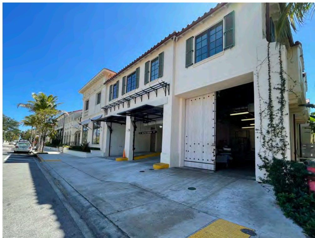
Rear, underground parking
