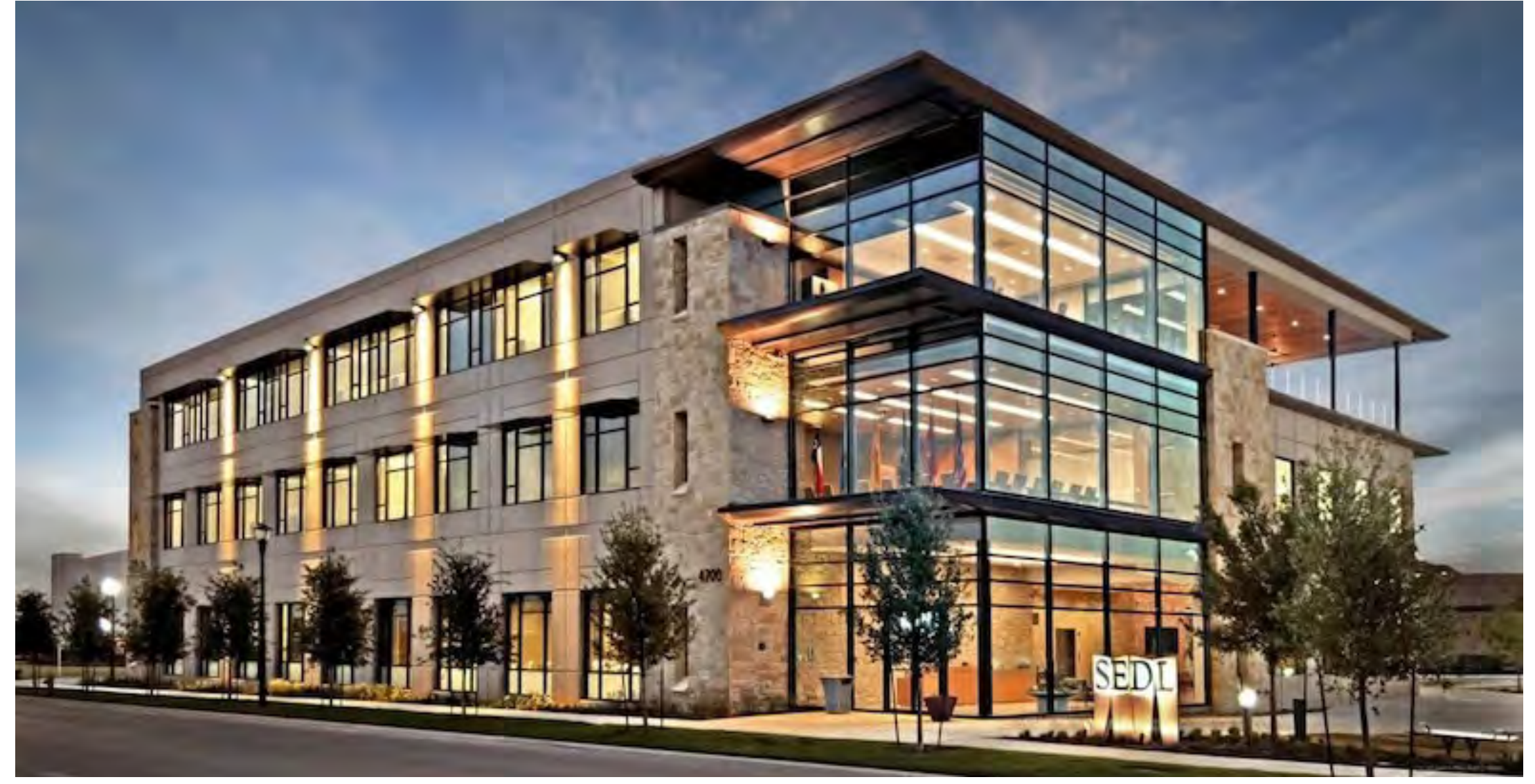
Large windows increase glazing and opens the transition between public and private spaces.
