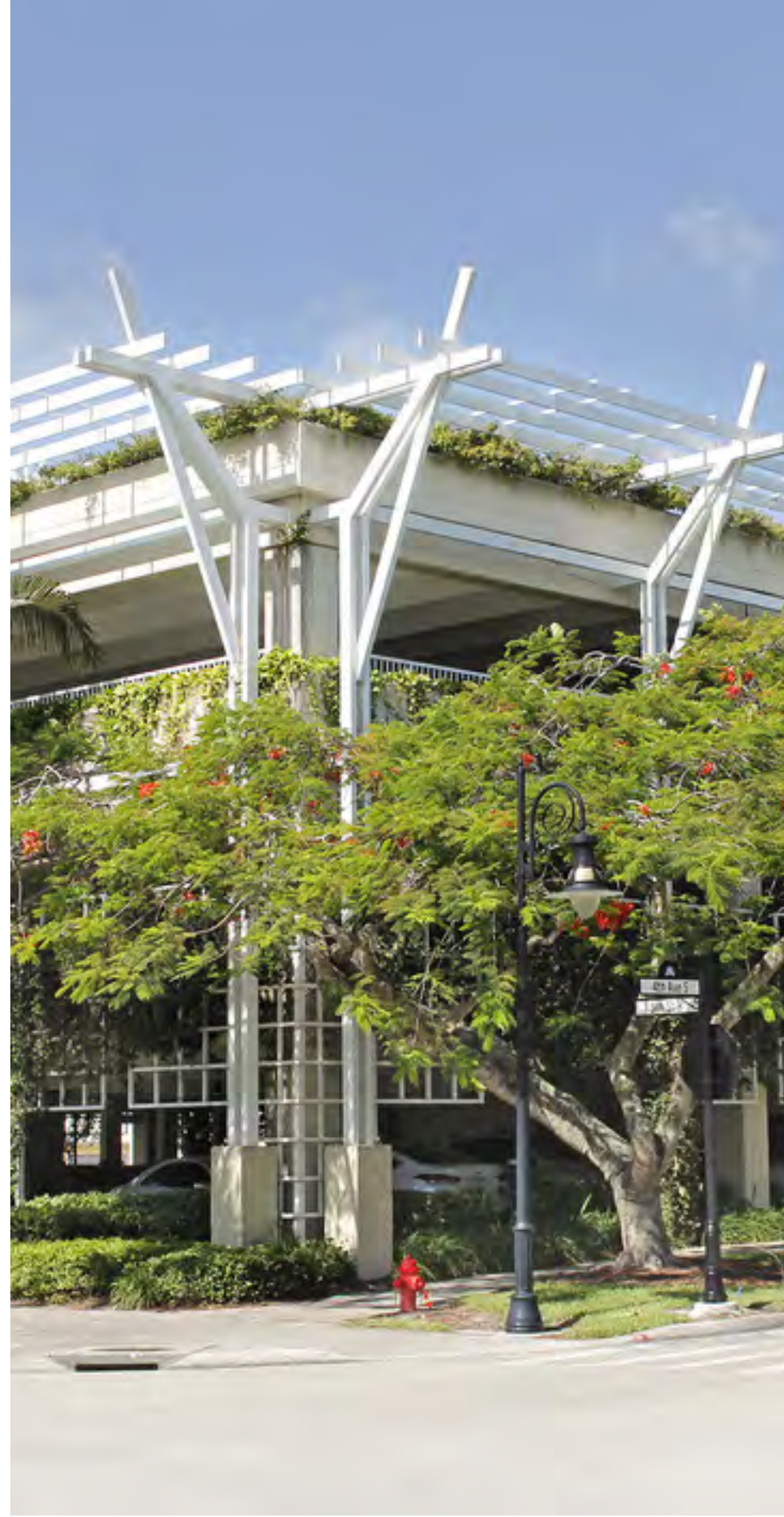
Parking garage screened by greenery.
