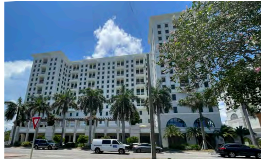
Trader Joe's Office Building on US 1 is a product of code allowing large footprints and setback exemptions.
