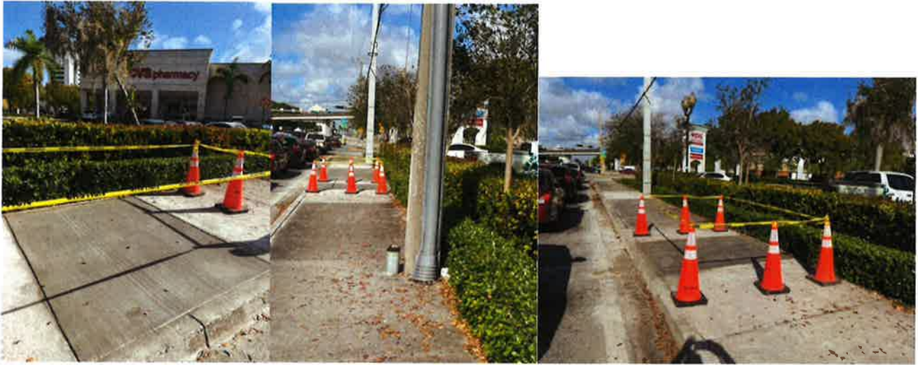
Coordinate with WASD to remove abandoned valve.
