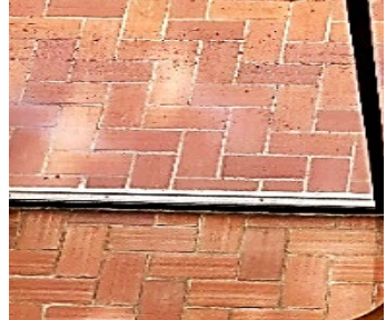
Unglazed clay tile flooring
