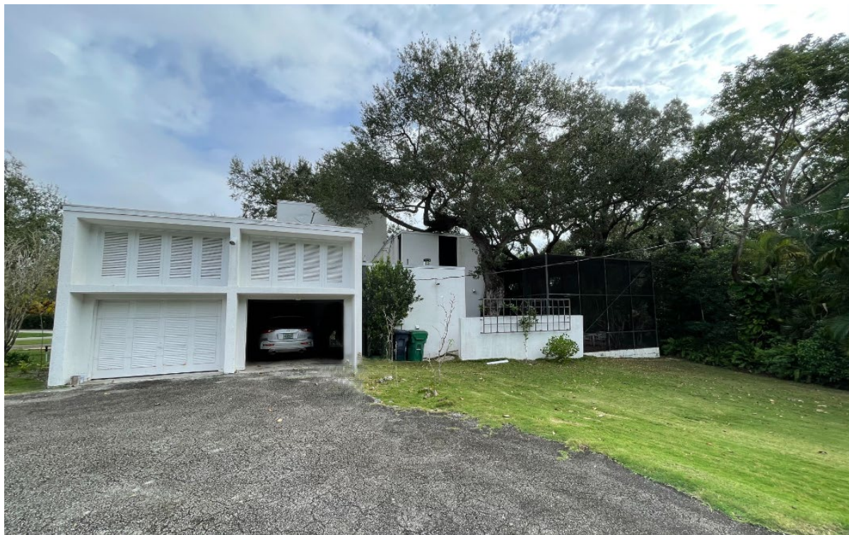
Garage at West façade with louvered doors 2024
