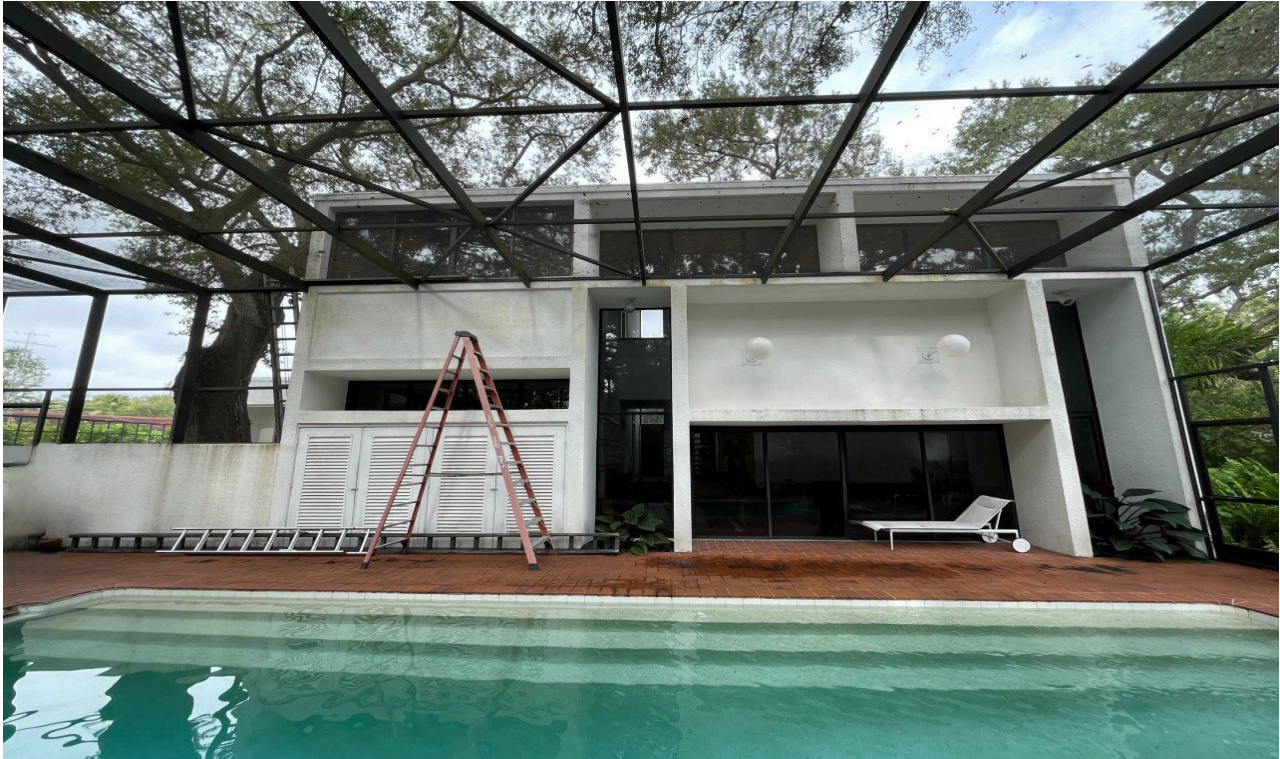
Screened pool deck at South façade 2024.
