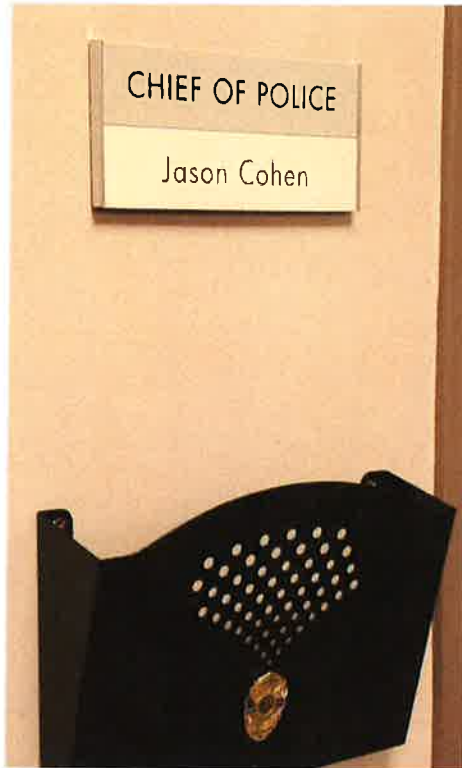
Installation of name plaques throughout PD
