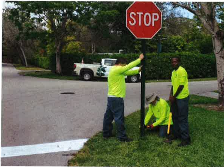
Installation of fallen stop sign and pole
