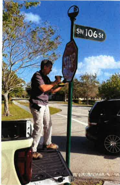
Installation of fallen stop sign
