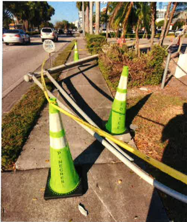
Create a safe area around pole and coordinate with FDOT for removal
