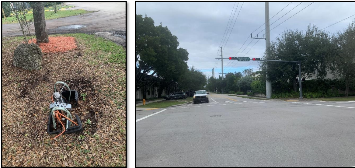
Figure 15 – Photos (left: exposed utilities; right: overhead transmission power lines)
