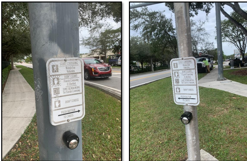
Figure 13 – Photos (faded pedestrian actuation sign at SW 124th Street)
