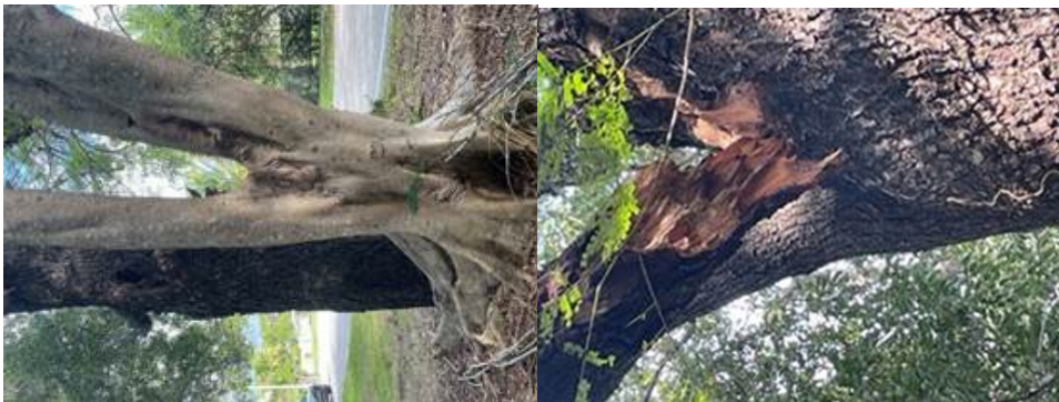
Branch removed hanging over sidewalk 77 th Ave between 133 rd St and 134 th street on the west side
