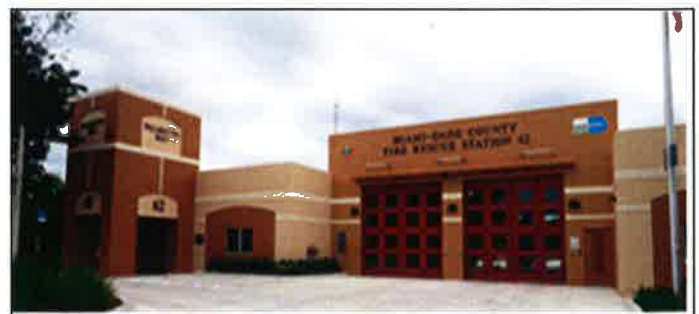
Palmetto Bay Fire-Rescue Station 62 serving the Village of Pinecrest
