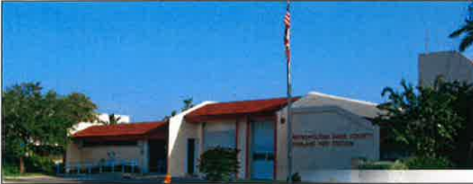
Suniland Fire-Rescue Station 23 serving the Village of Pinecrest
